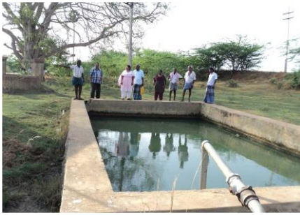
Sump Constructed at Senkulam Tank to use water for irrigation
